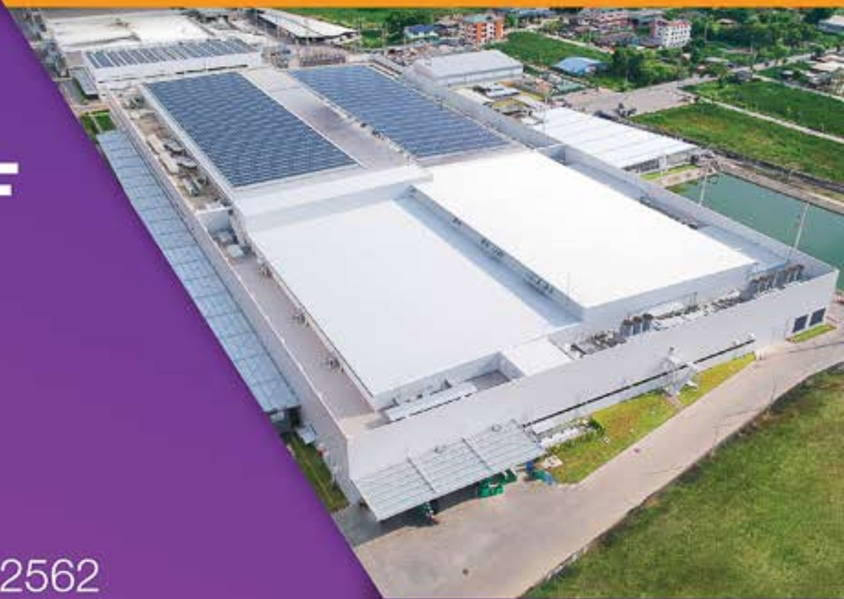
▼ Lamp 7 Extension Factory
